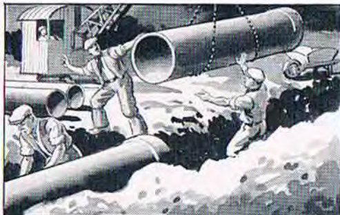
Bad sanitation means bad health. In 1851 the city took over complete control of sanitation. Now there are nearly 1,400 miles of sewers.
