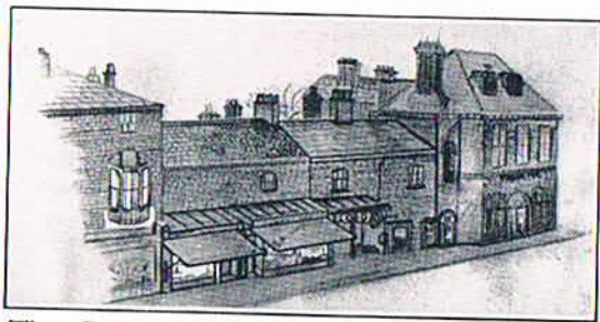
This Drawing was made from the window of the classroom. It shows how new shop fronts have been built on to the fronts of ordinary dwelling houses.
